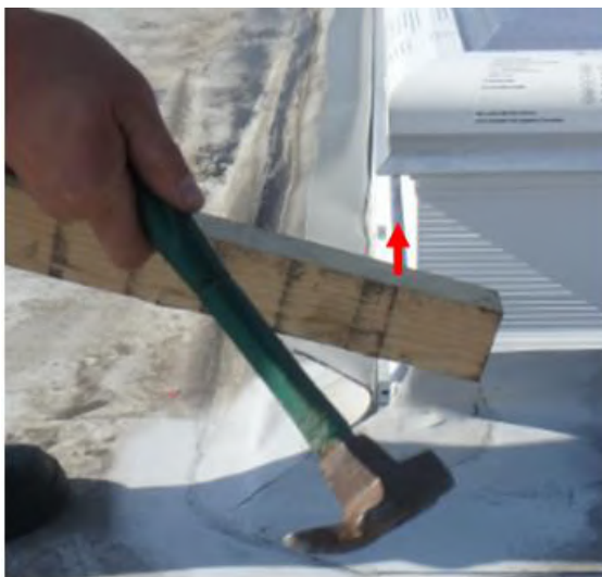
Fig. 19. Driving the connector.
