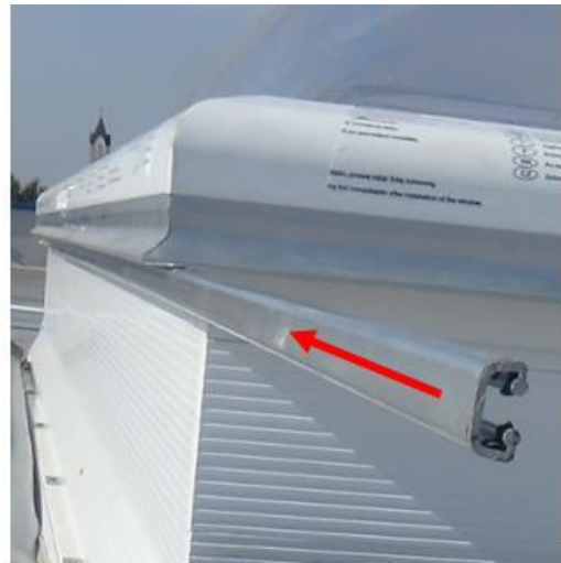
Fig. 18. Sliding the connector.
