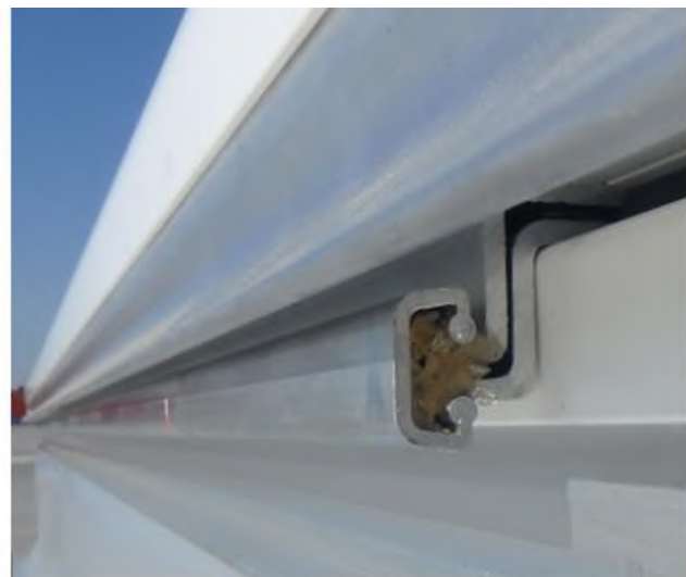
Fig. 20. Hinge with fitted connector.
